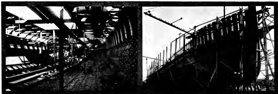
Interior and exterior views of the big wooden steamer being built at the Kiernan & Kern Shipbuilding Company's plant at Portland, Ore.
